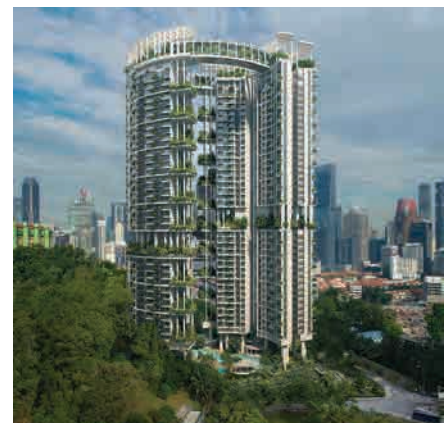
ALL IMAGES: One Pearl Bank will have 39-storey towers linked at the roof by sky bridges, plus a series of sky allotment gardens .
