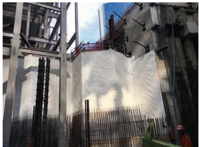
ALL IMAGES: Preprufe Plus waterproofing membranes from GCP Applied Technologies have been selected for use in the Commercial Bay project in Auckland, New Zealand, to protect its basement and transport connection link.
