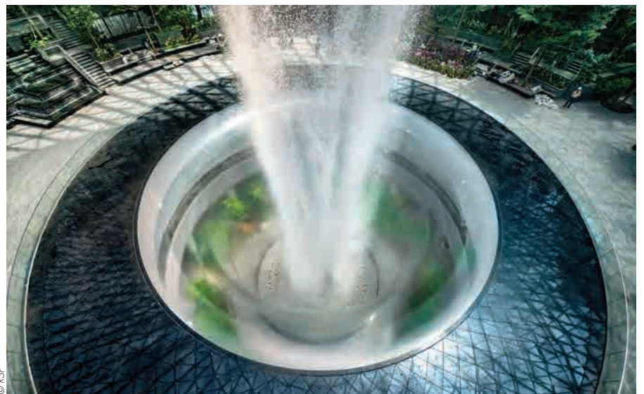
TOP AND ABOVE: More than 10,000 gallons of water reportedly flows through the oculus per minute at peak conditions.
