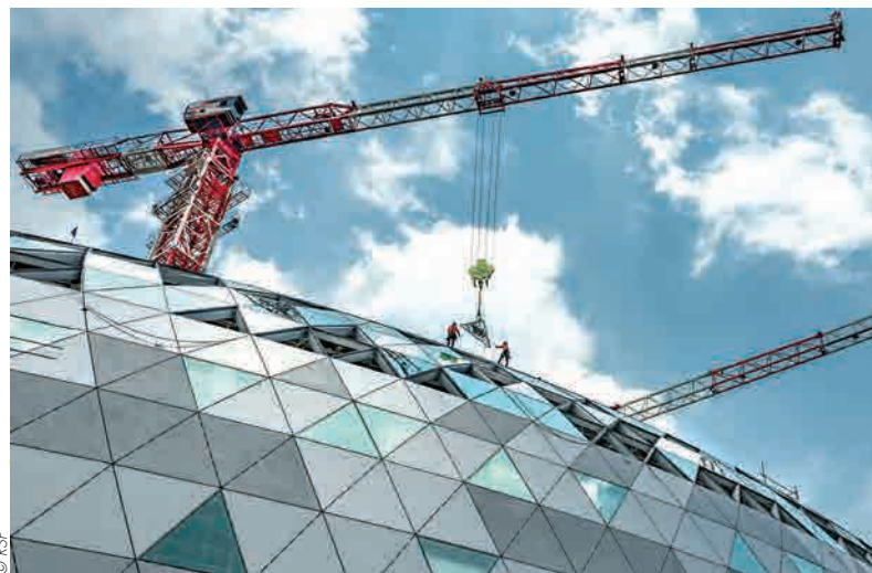
TOP, ABOVE AND ABOVE LEFT: The installation of the dome-shaped facade posed a major challenge to the project team. It required more than 9,000 glass panels, about 18,000 steel beams and over 6,000 steel nodes.
