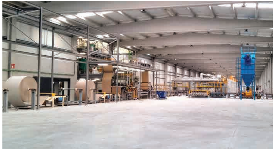
MMM Erba Makina's gypsum plasterboard plant.
