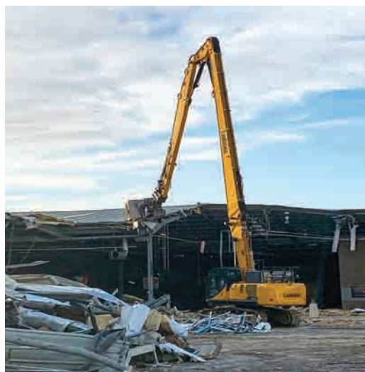
LEFT: LiuGong 950 demolition excavator.
