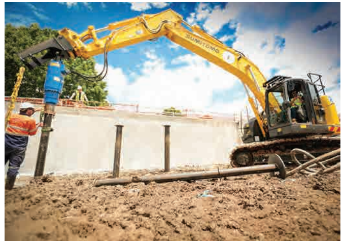
ABOVE AND LEFT: Auger Torque 100,000MAX earth drill is designed for excavators up to 50 t.
