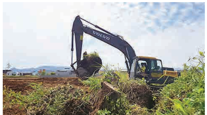
TOP, MIDDLE AND ABOVE: Volvo EC200D helps Indonesian developer PT Bumi Mapanget Asri to build a 300-ha housing complex in Manado. The machine is currently preparing the land for the first phase of construction.
